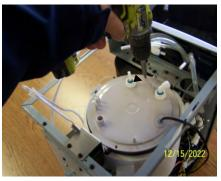
4.11 Remove top/Purechill assembly from cold tank
