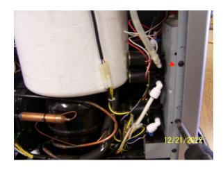
7.6 Pull mounting plate out to access solenoids
